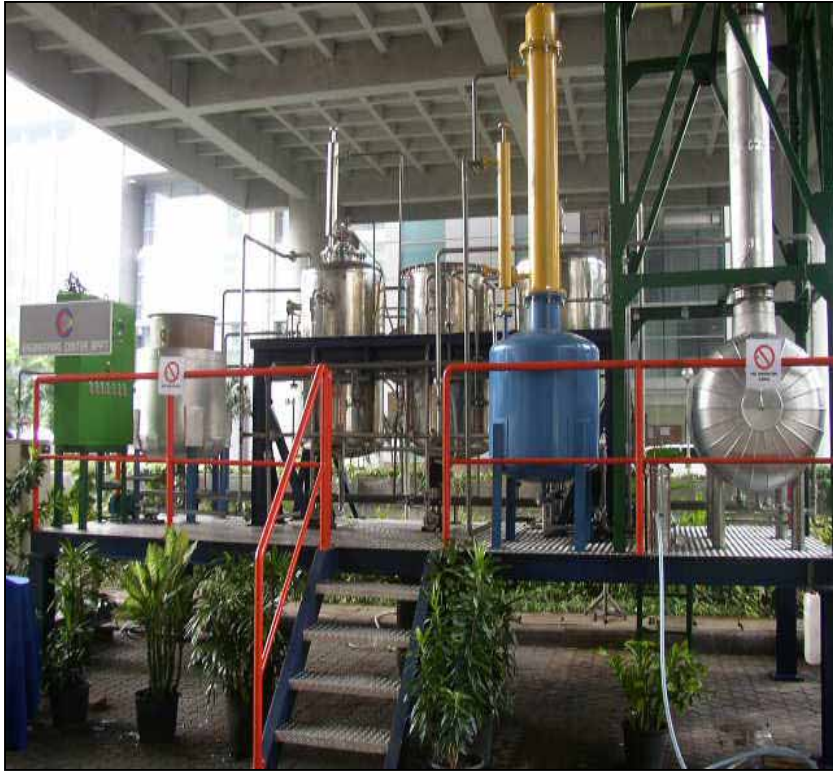
1.5 Tons/day Prototype Biodiesel Plant
