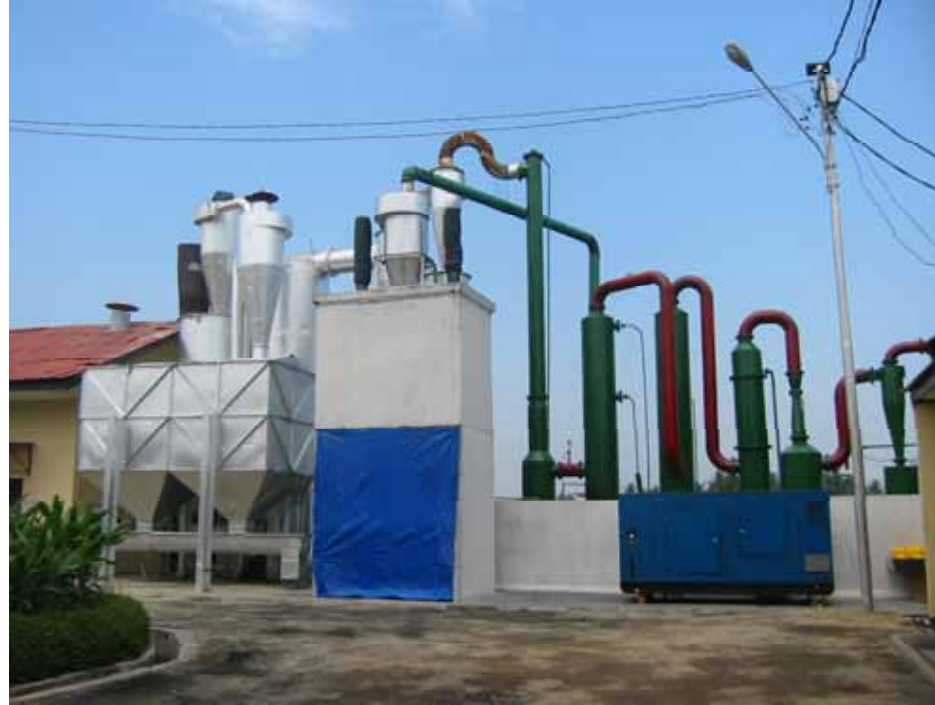
Rice husk gasifier for electric generator (0.5 MW)
