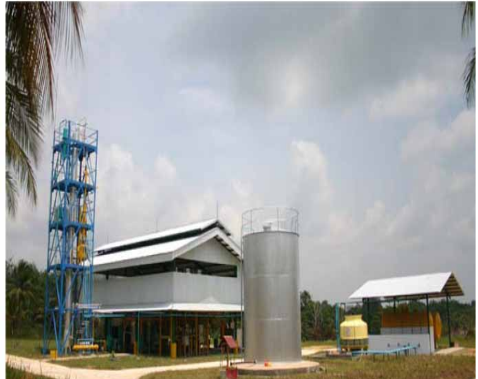
8 Tons/day Prototype Biodiesel Plant
