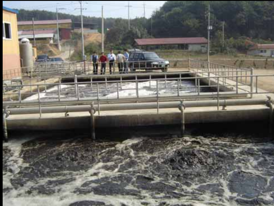
Animal liquid manure purification with active sludge
