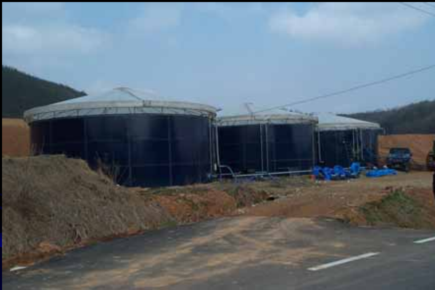
Liquid manure storage container 1) Capacity : 200 ~ 500 m 3
