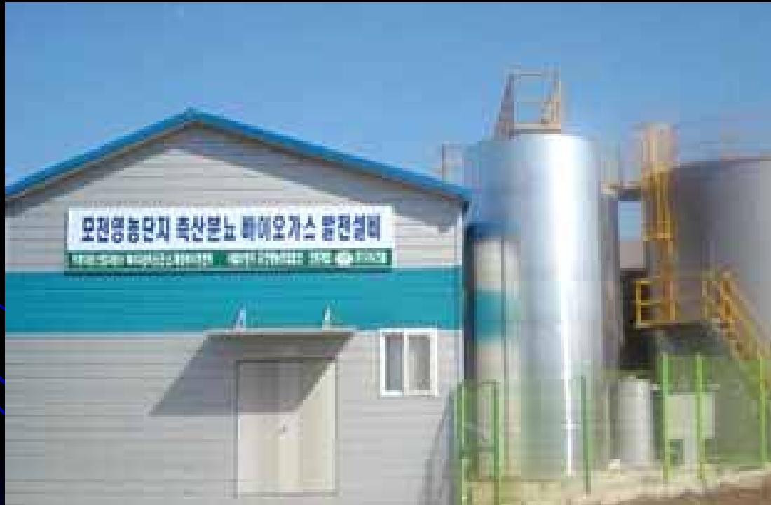
bio-gas electricity generation plant
