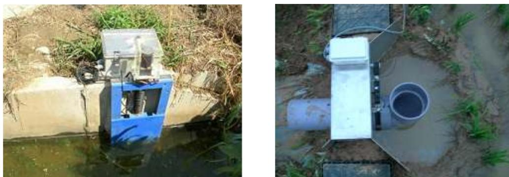
Fig.12. Automatic type inlet (left) and outlet (right).
