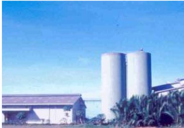
Figure 1. Typical concrete tower silo storage systems with and without out roof
