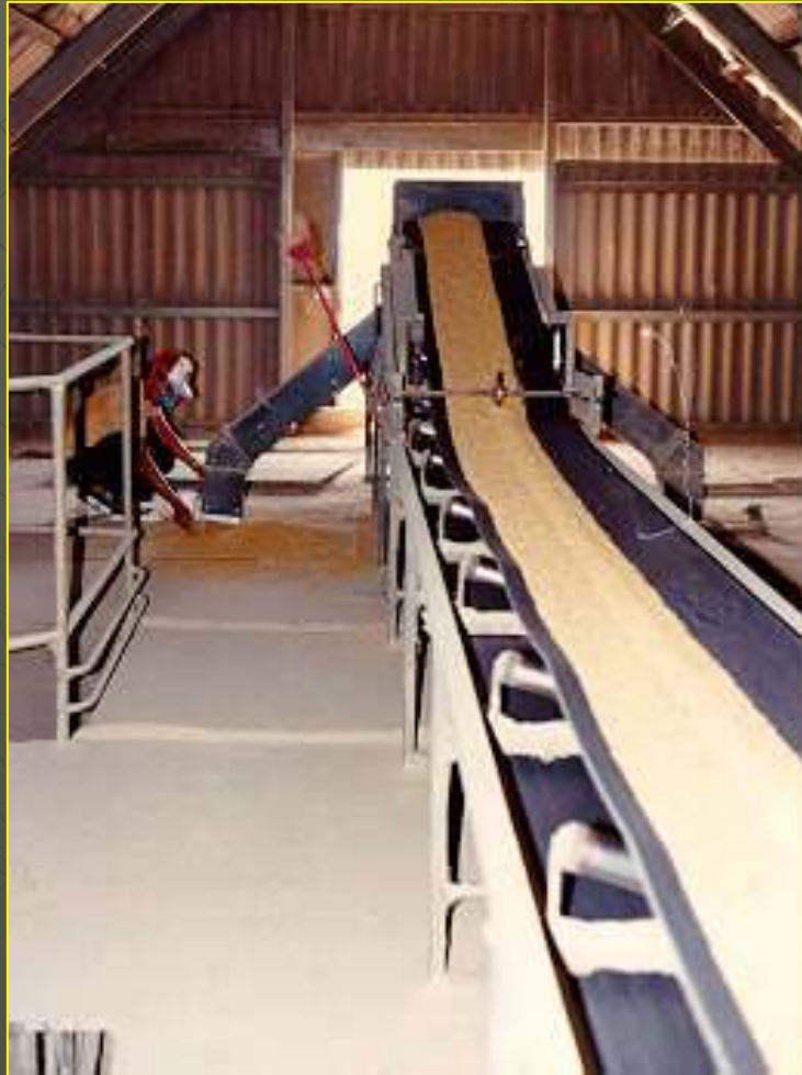
Loading of dry paddy into the silo
