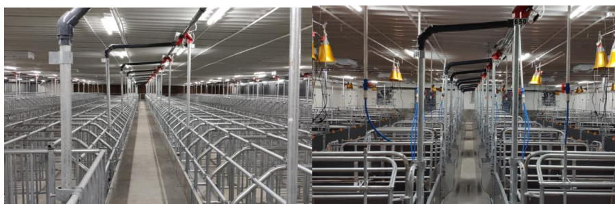
(a) Wet feed feeding system of distribution room (b) Wet feeding system of delivery room
