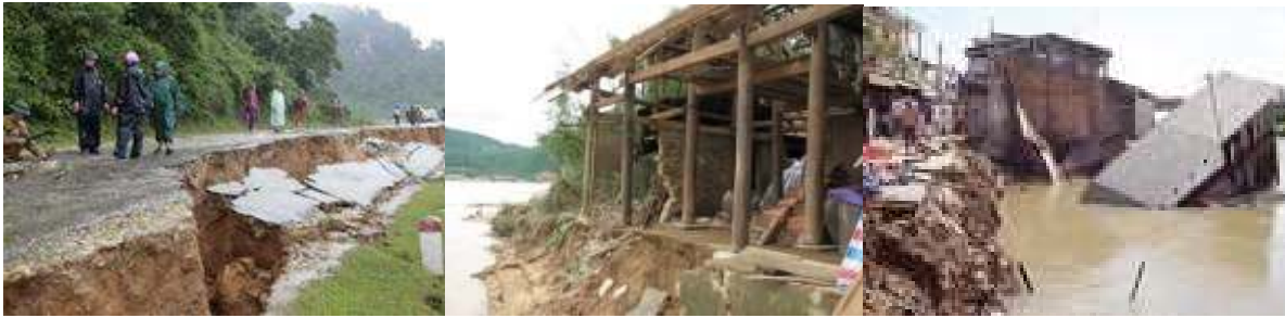
Figure 6- Typhoon and flood destroy crops, seeds and fertilizers, riverside collapse
