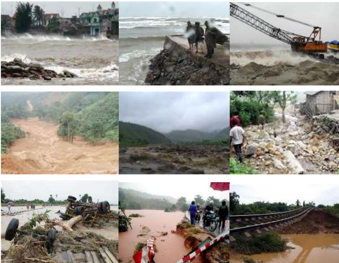
Figure 7- Typhoon and flood destroy dykes system, soil erosion, constructions and transport
