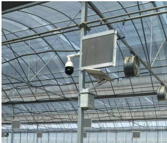
大棚环境监测设备 Environmental monitoring equipment for greenhouses
