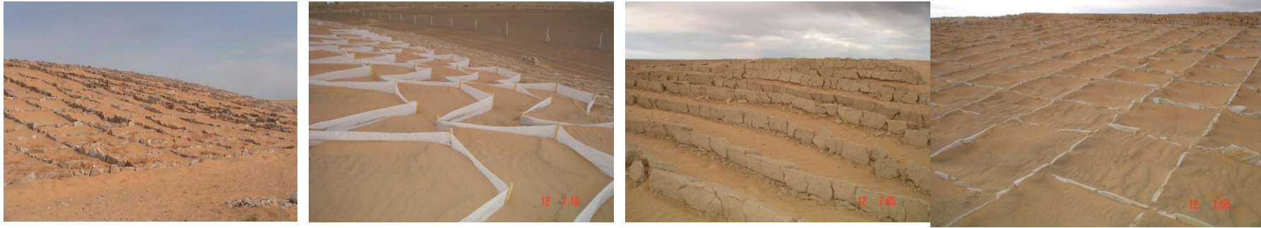
Mechanical techniques using stones, clays, and nets implemented in Umnugovi province for the purpose of abating sand movement.
