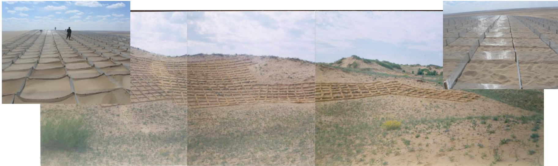
Mechanical techniques using straws and nets implemented in Tuv and Dornogovi province
